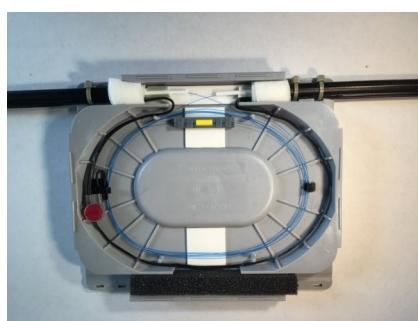
Trim excess tracer/toner wire and splice with suitable connector. Route tracer/toner wire and secure under fence with clip using care not to disturb or damage fiber. Toner wire and connector should be adjusted to be flush to base.
