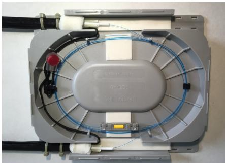
Wind the fiber ends into the base in an oval pattern in the race track, keeping the fibers between the fences to determine where the fibers will meet to be spliced.
