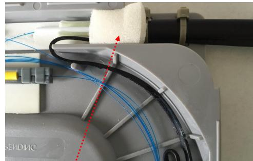
Wrap the cable end once or twice with the foam wrap. For smaller diameter cables, cut or tear at least 1" length of foam bar and place on top of cable over the foam wrap before installing the cover. Align the end of the strength members with the end of the interior wall as shown. Secure cable using cable ties. Hint: When inserting the wire tie, start by inserting the wire tie in the outside slot from the top, keeping the wire tie head on the top so that the kit lays flat for proper filling.
